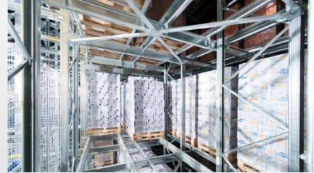
Channel storage deep-freeze HBW
