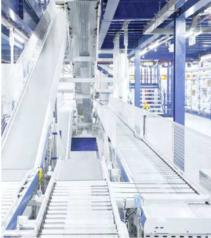
Long-span shelvings caters for slower-moving items at the 2nd-3rd floor
