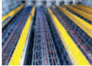
Storage and Retrieval Systems
