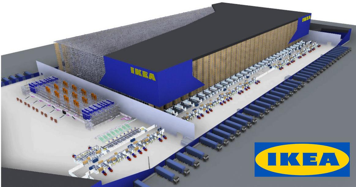
IKEA selected SSI SCHAEFER for the implementation. Core elements include an automatic shuttle warehouse design that utilizes the **SSI SCHAEFER 3D-MATRIX Solution**<sup>®</sup>, a high-bay warehouse (HBW) with 245,000 pallet storage locations, ergonomic multi-order-picking workstations, and the warehouse control software—**WAMAS**<sup>®</sup>.
