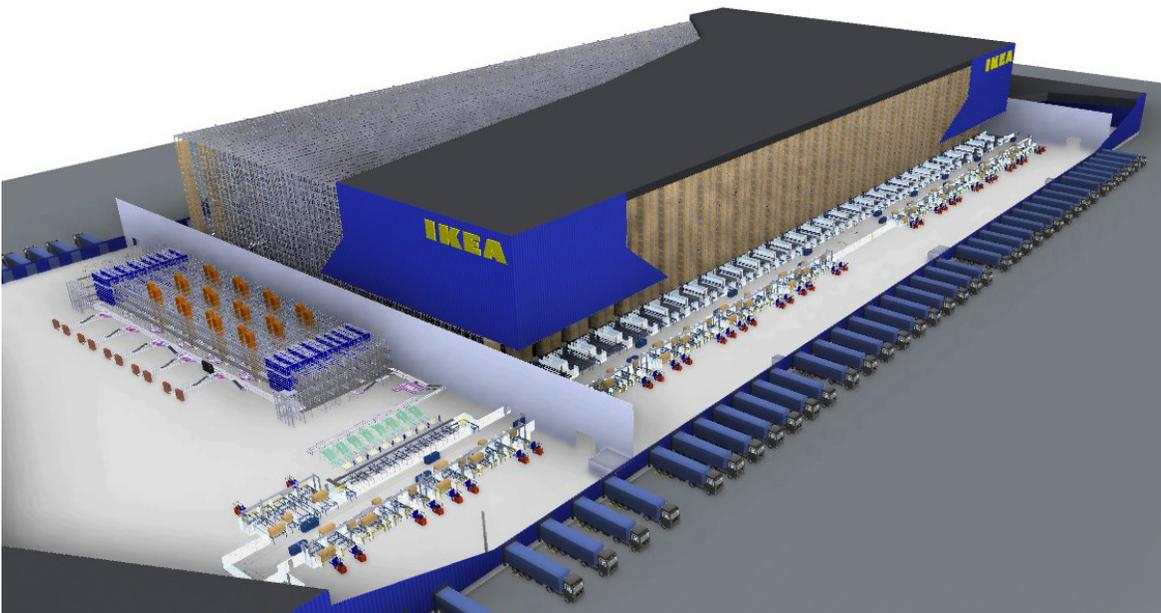
Ikea selected SSI SCHAEFER for the implementation. Core elements include an automatic shuttle warehouse design that utilizes the **SSI SCHAEFER 3D-MATRIX Solution®**, a high-bay warehouse (HBW) with 245,000 pallet storage locations, ergonomic multi-order-picking workstations, and the warehouse control software—**WAMAS®**.
