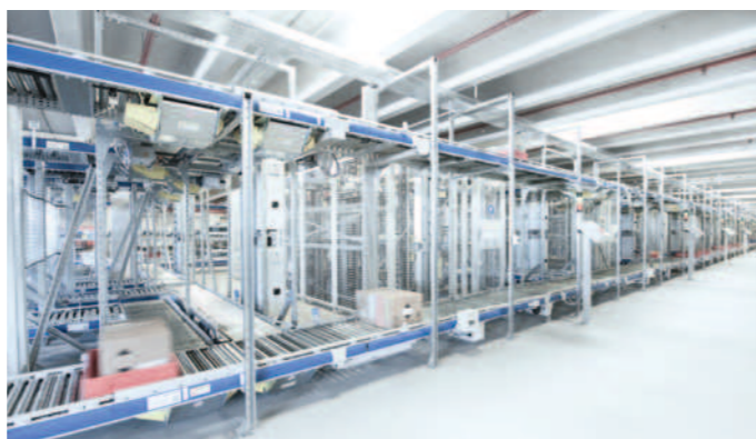
Connecting conveying system of the miniload from goods-in to the picking and shipping locations
