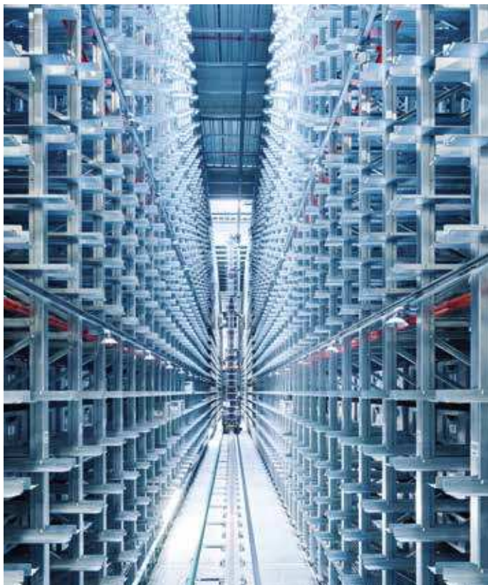
Two-story automated miniloads with Schäfer Miniload Cranes
