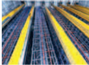
Storage and Retrieval Systems
