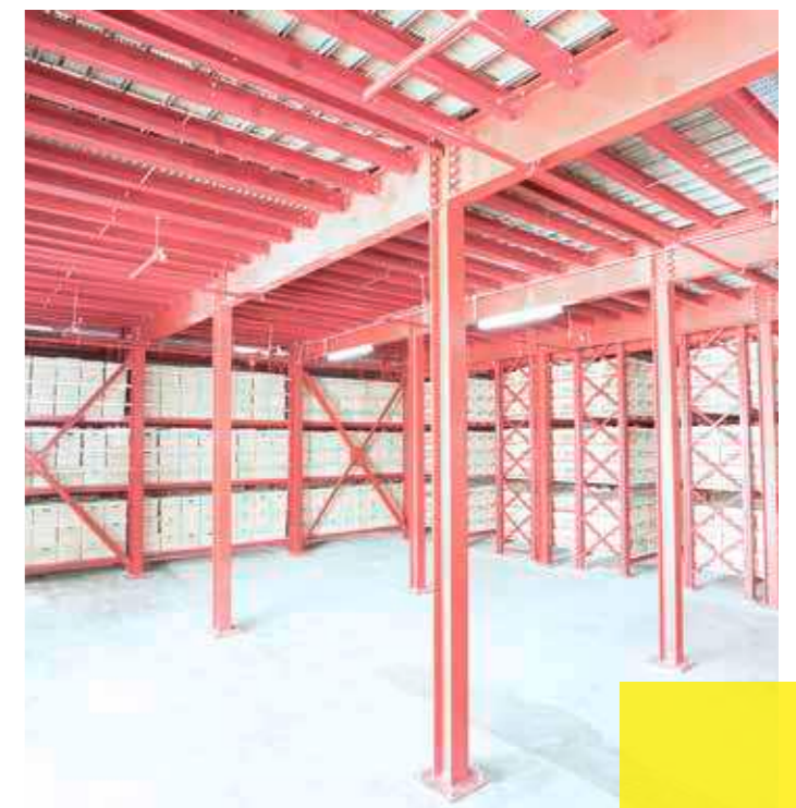
Mono-post beams create additional area for workspace and storage
